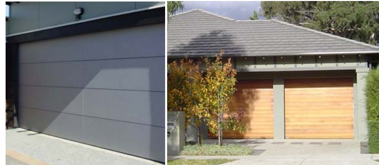
Double garage doors should consist of double tilt up doors (left) or two single doors separated by a 300mm column (right)
